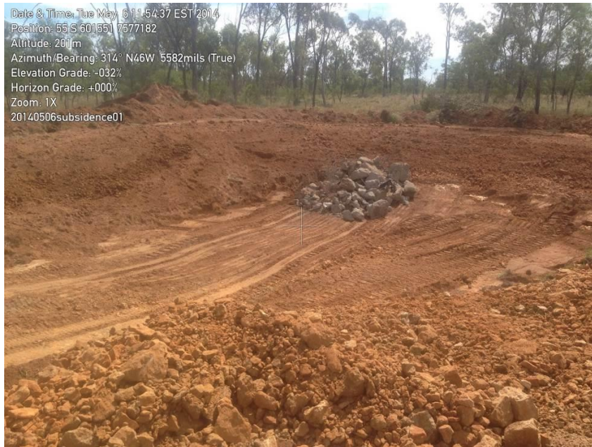
Figure 4 - Placing clean fill in an excavated subsidence crack
