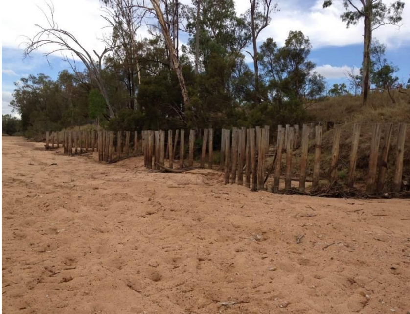
Figure 7 - Completed pile fields at Moranbah North Mine
