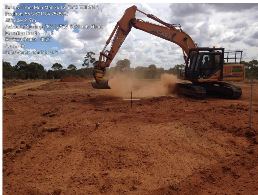
Figure 5 - Replacing topsoil over the treated subsidence cracks
